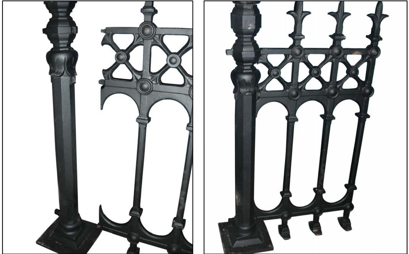
Intermediate post and Stewart railing section
