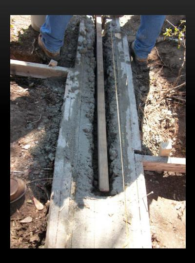
This creates a slot for the root fixing legs of the fence to fit into. Depending on your style of fence, the slot may need to be deeper or your footing contractor may pour the entire footing around the fence panels
