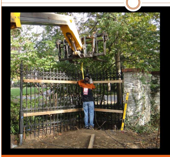
Fully welded panels are easy to handle by light cranes or lifts and allows for quick installation by 2-3 workers.
