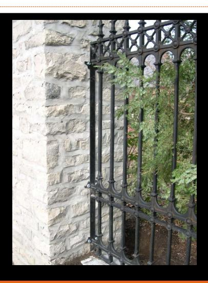
Fence Panels are trimmed where they meet the masonry columns and small custom clips are added and welded to accept attachment of masonry anchors.
