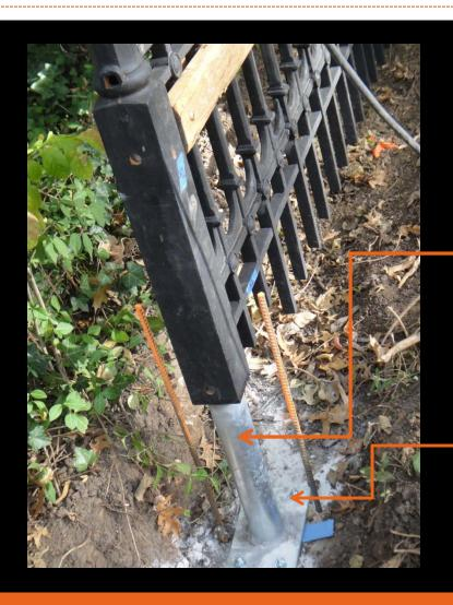
Once the posts are located, a continuous trench footing was poured under the fence line and the post locations were enlarged and reinforced.
